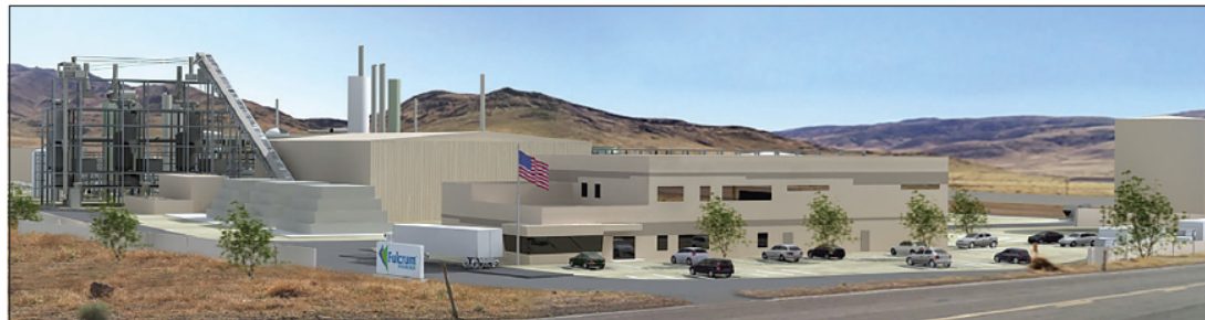
Fulcrum has started construction of its first commercial plant outside of Reno, Nevada, and is advancing on the development of additional plants across North America with the capacity to produce more than 300 million gallons of jet fuel and diesel annually.
